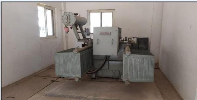
Figure 3: Indoor 11/0.415 kV (800 kVA) Transformer
