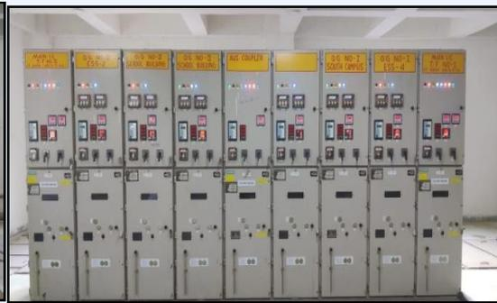
Figure 2: 11 kV Distribution panel
